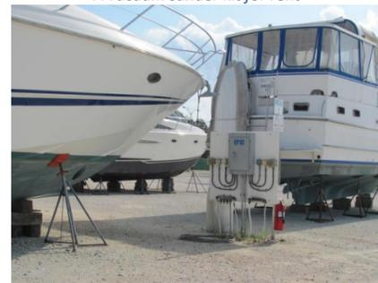
Air, power, and water panels are located at each working stall.
